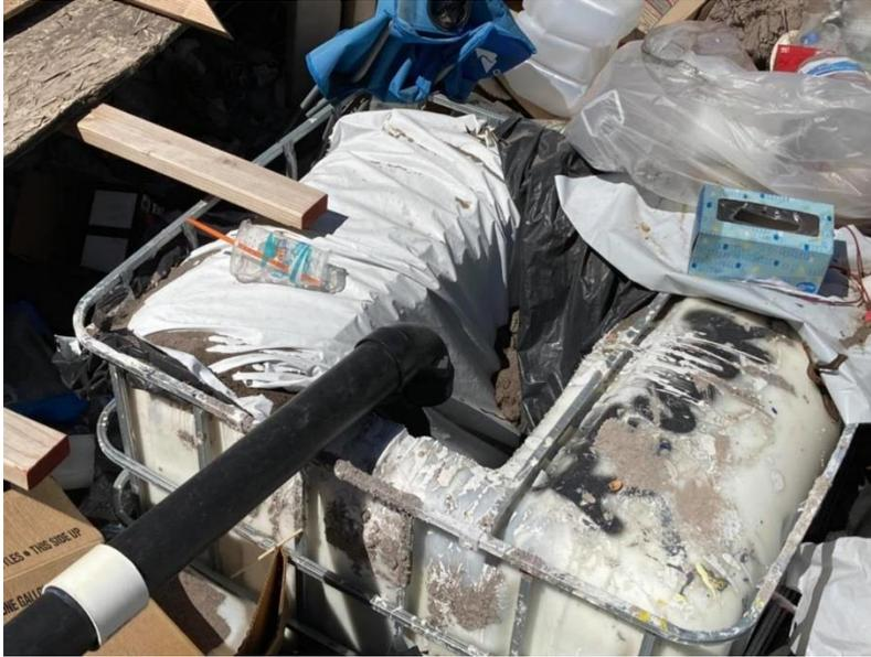
250-gallon caged water container used as an illegal sewage septic system.
