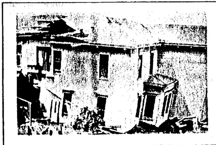
House built across fault at Wright's Station. 1906 earthquake.
