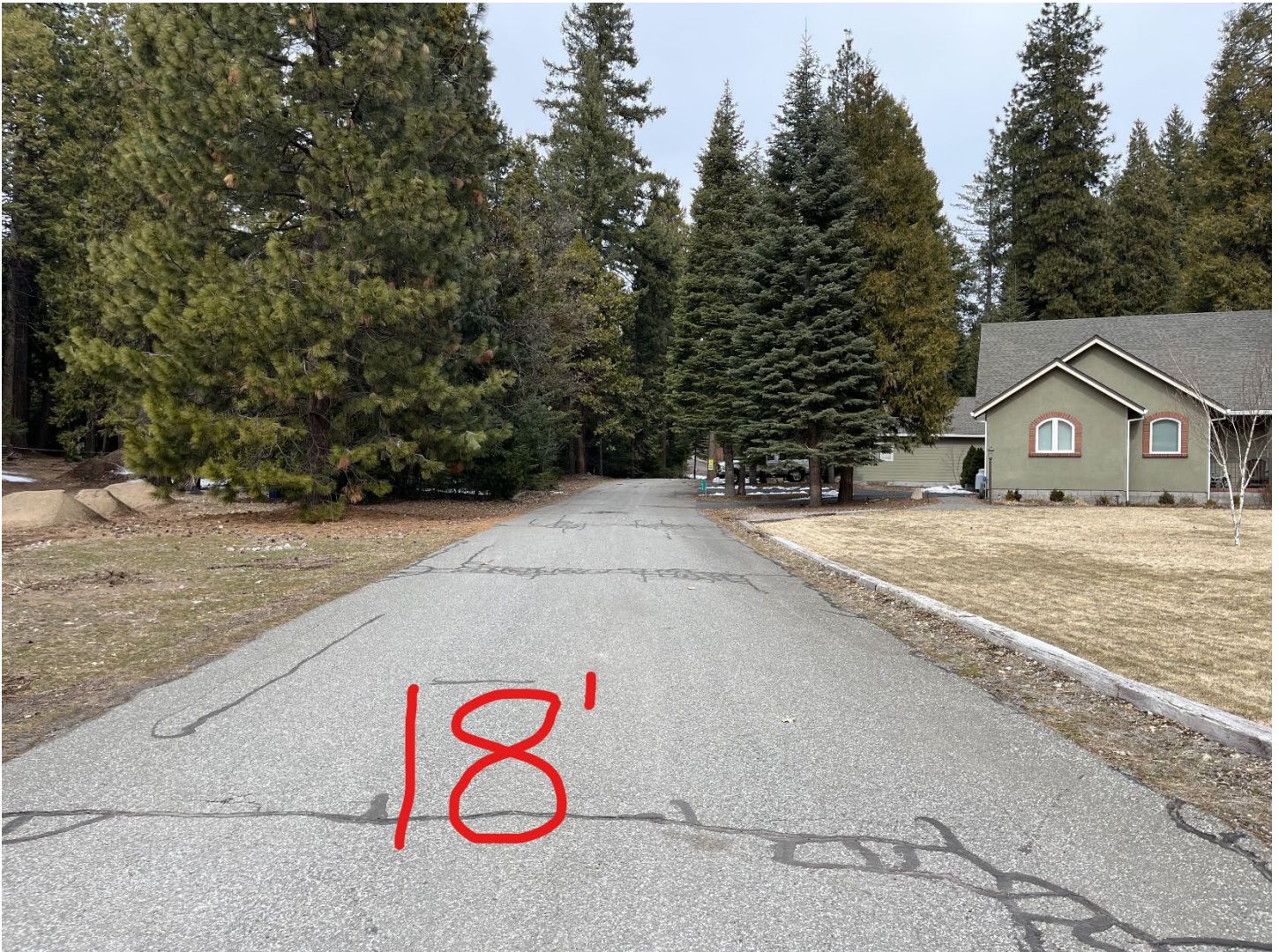
Figure 2: Paved portion of Laura Marie Lane measuring approximately 18' in width.
