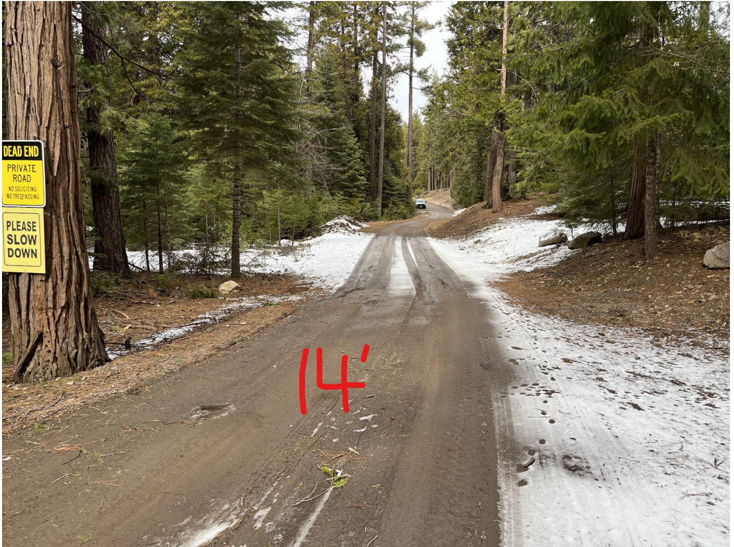
Figure 3: Traffic lane at this point measured approximately 14' in width.
