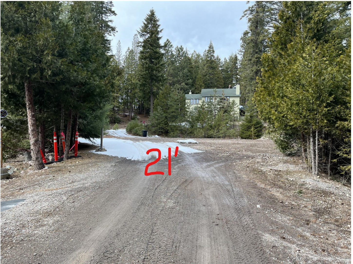
Figure 4: Traffic lane at the entrance to applicant's property measured approximately 21' in width.
