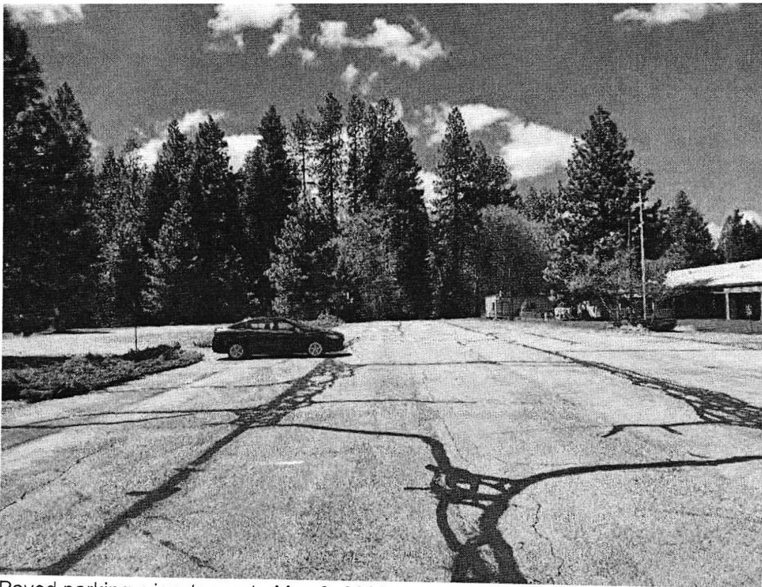
Paved parking, view to west. May 3, 2023.
